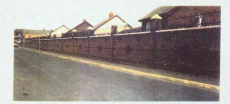
1m Crook-Arm Metal Railing Mounted on 2.4m Brick V
