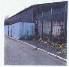
2.5 High Profile Steel Cladding mounted on 2.5 High Block Wall
