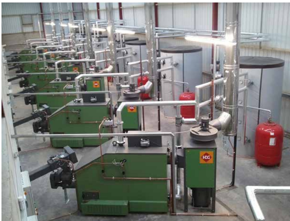
Figure 6 – A Multiple Boiler Installation
